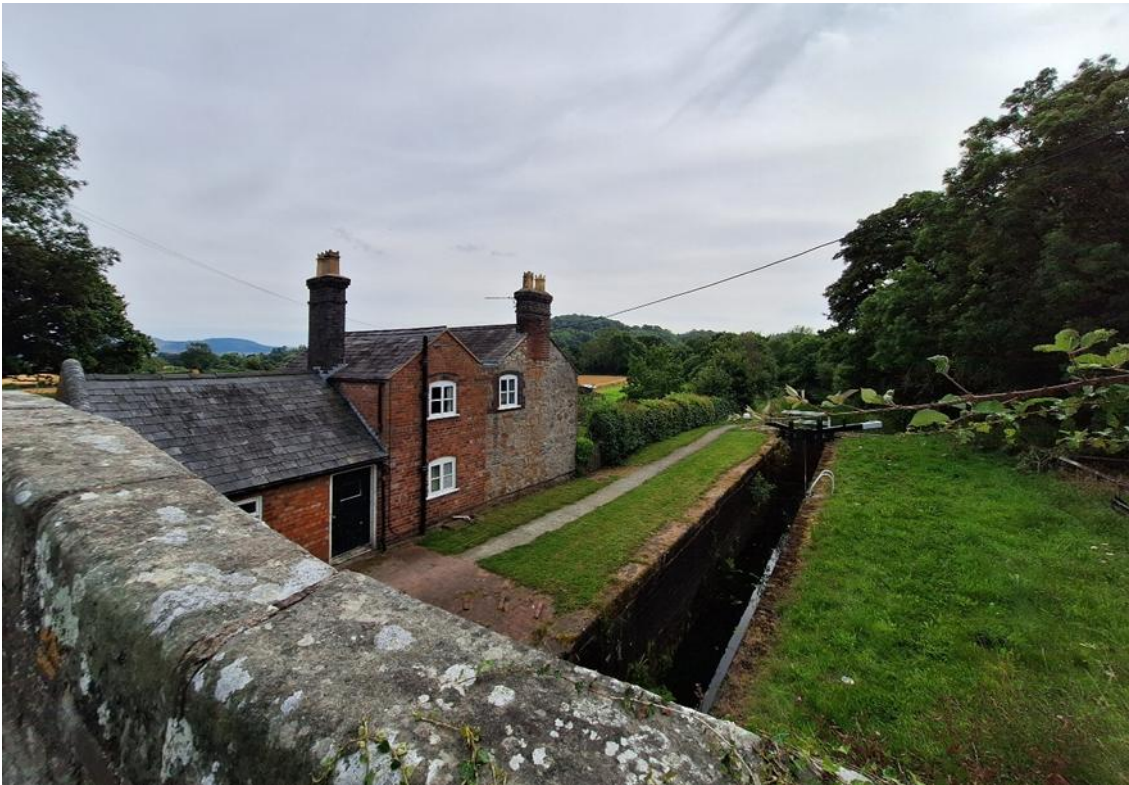
Figure A9.1.22 – View looking Southwest from Bridge 95 (Cadw Ref. 14187) towards the Lockkeeper's Cottage (Cadw Ref. 14189) and the Lower Lock chamber (Cadw Ref. 14190)
